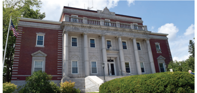
The Hancock County Courthouse will be returned to the County when a new courthouse is built.
